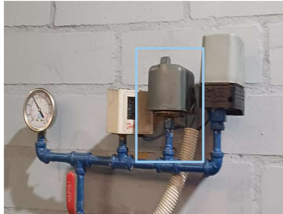
**Figura 6.** Presostato a reponer.
